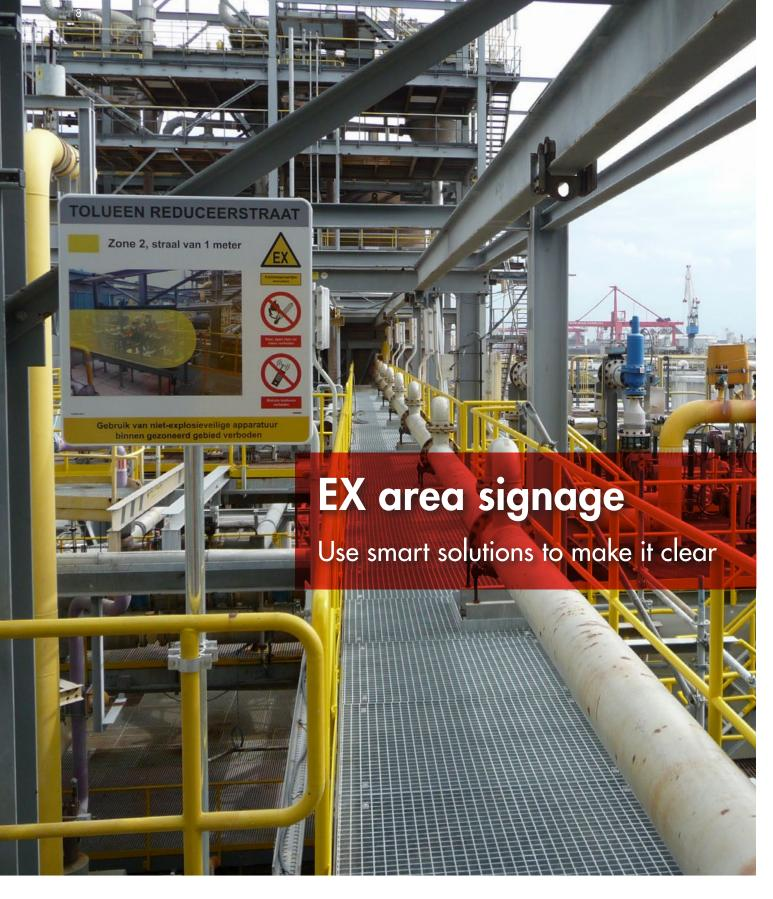
Indicating explosion hazardous areas is not always straightforward: simply applying the safety symbol may not provide enough information in many cases. Using photo-impression boards, for example, makes it possible to give a clear picture of the explosion hazard areas. To delimit the zone even more clearly, markings and cordons can be used in addition to the signage – a practical implementation that is aimed at being fully clear to whoever sees it.
